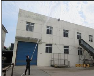
External photo(s) of the production unit(s) functional fire hydrant.JPG
