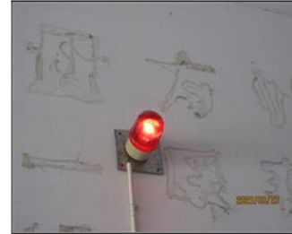
External photo(s) of the production unit(s) functional fire alarm.JPG
