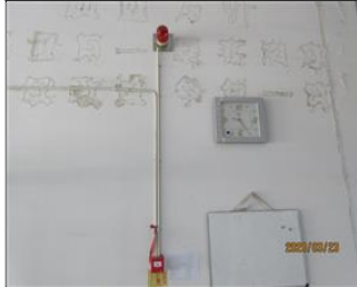
External photo(s) of the production unit(s) fire alarm and button.JPG
