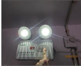
External photo(s) of the production unit(s) functional emergency light.JPG
