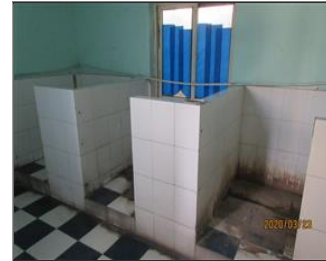
External photo(s) of the production unit(s) Finding 7.22 no privacy door for the toilet.JPG
