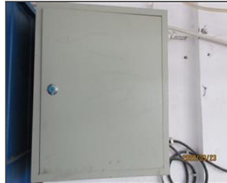
External photo(s) of the production unit(s) Finding 7.9 no warning sign for electrical danger.JPG
