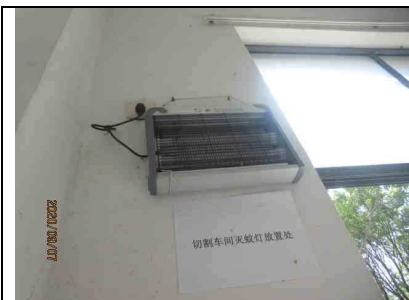
25) One set of fly kill lamp installed at cutting workshop was not working properly
