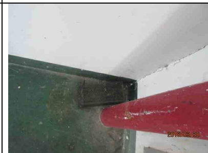
41) Mouse trap equipped in gluing workshop was not in working condition
